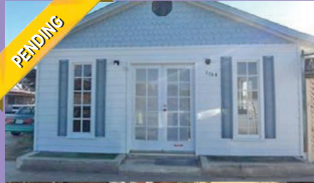
374 Pier Ave., Oceano. Charming Duplex located steps to the beach. Many possibilities with this property. Currently the back 2 bedroom is being rented. Mirrored front unit can be used as a business. Check with county as to property uses. Property is located at the entrance to Oceano Dunes.
